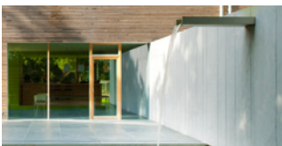
60 woningen in Kalmthout
